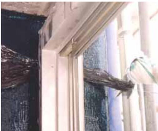
(a) The CF-anchor under installation
